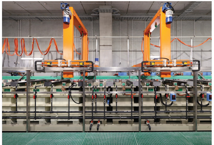
Allegion New Zealand's leading edge automated electroplating plant.
